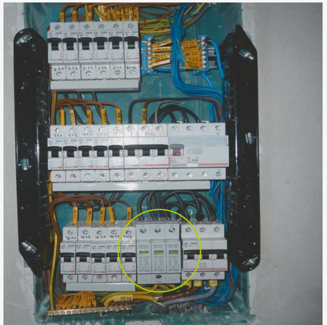
Switchboard cabinet after the the SPD is correctly installed.
